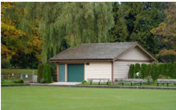
New Machine Shed Built
