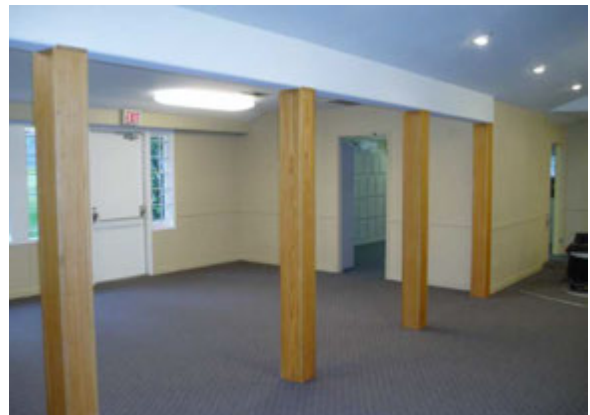
Renovating the Clubhouse - Replacing the wall to the back room with beam and posts. Dave Hinds (lower left) was the carpenter in charge of this project. The carpets and lights were changed and the interior painted. Note the finished product (lower right).
