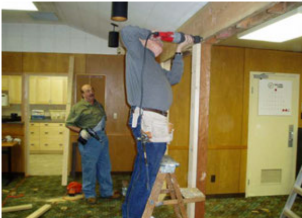
Renovating the Clubhouse - Replacing the wall to the back room with beam and posts. Dave Hinds (lower left) was the carpenter in charge of this project. The carpets and lights were changed and the interior painted. Note the finished product (lower right).
